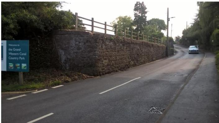
It is expected to take nine weeks to remove the existing wall, dig out the tons of earth behind it, build a new retaining wall, and to create the new pavement. A temporary telegraph pole has been installed to preserve the power supply to the Duck's Ditty floating café-bar whilst the underground cables are disconnected. The new concrete wall will be faced with stone from the existing wall so that the historic
